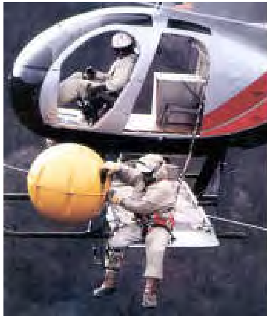
Figure 31. SpanGUARD Installation [29]
