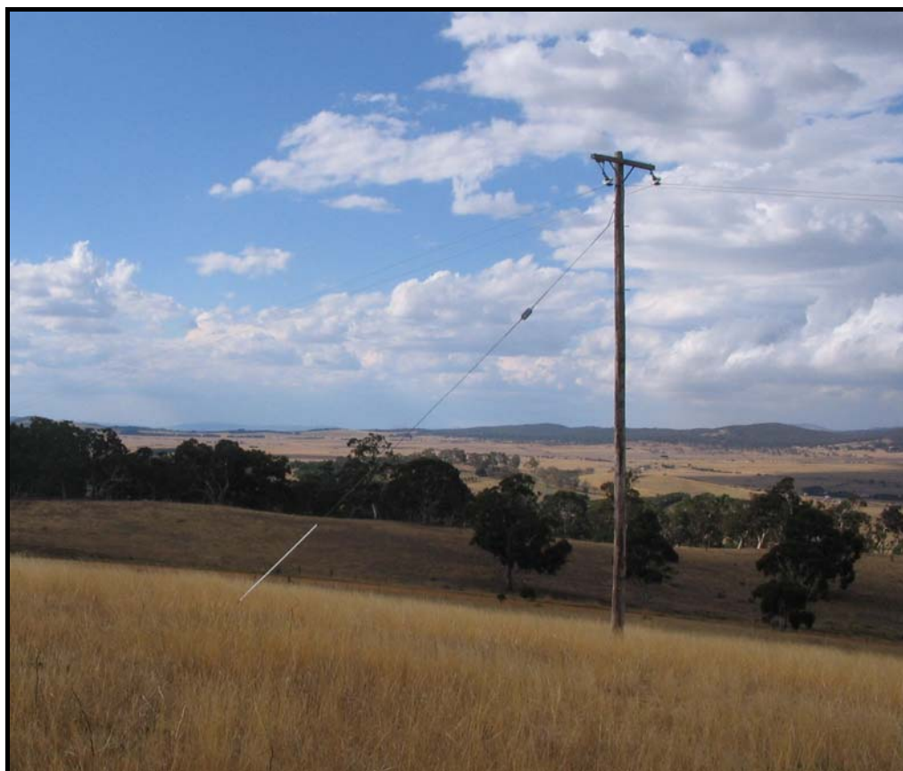
Figure 18. Example of a guy wire
