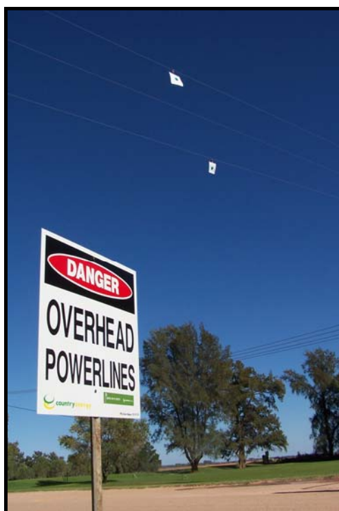
Figure 25. Example of a 'flag marker' used on overhead powerlines
