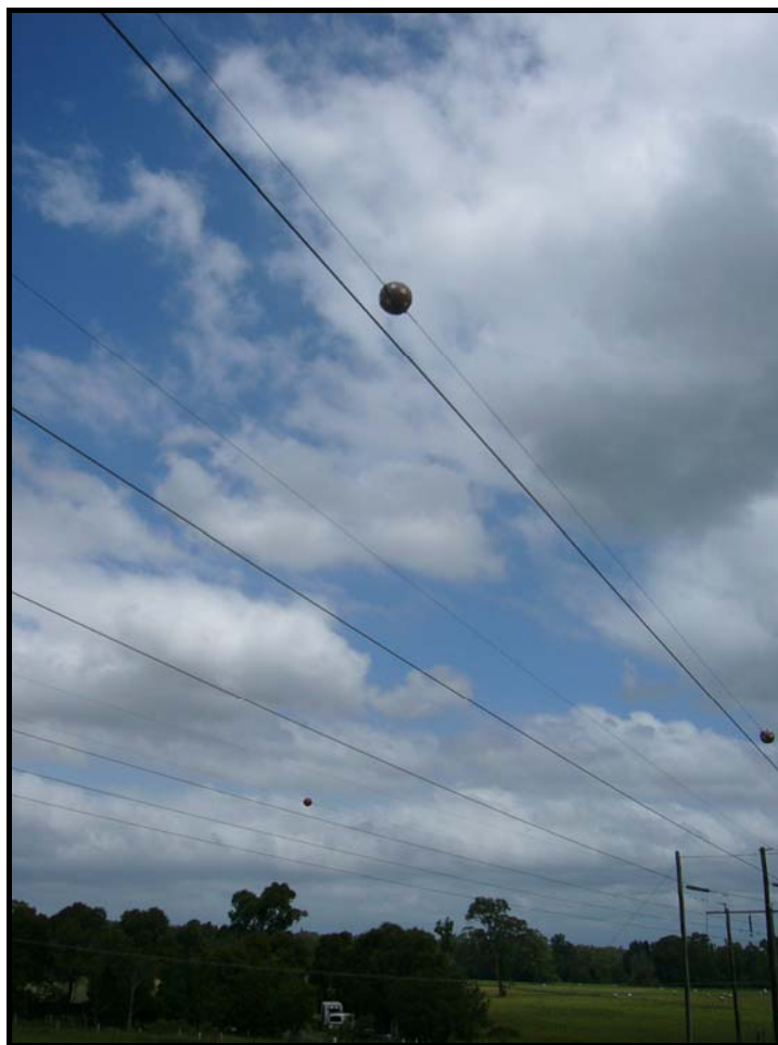
Figure 23. Example of wire markers mounted on a multi-strand powerline
